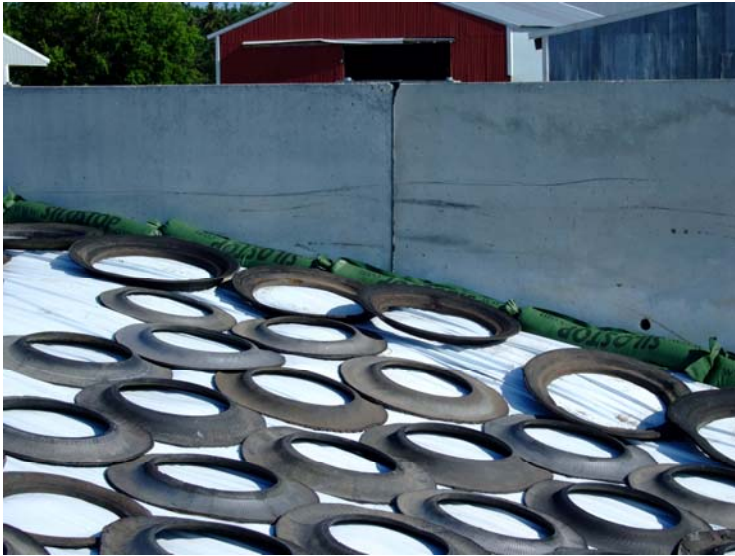
Figure 1. Gravel bags at the wall in a bunker silo.
