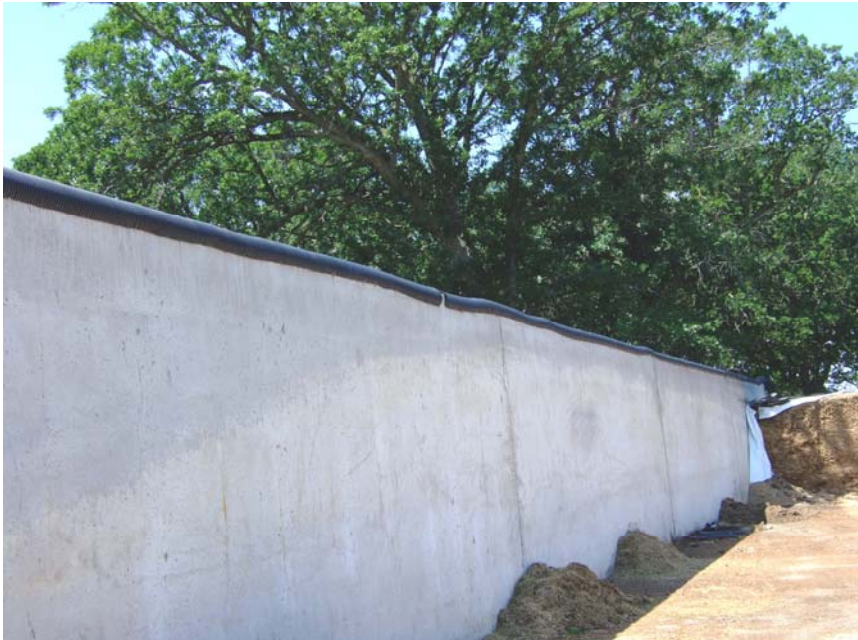
Figure 2. Plastic drain pipe used to cover the top of the wall to prevent side wall plastic from being torn or punctured.
